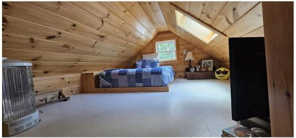
The above picture is of a loft in a newly added addition to the building below. This was created by a retired fire chief. This doesn't meet code in any fashion as this doesn't qualify as a Tiny Home in Maine. Doesn't have thew required head room, no smoke detector and has an unvented gas heater in a sleeping area,. This property is listed on a short-term rental site. It poses a danger to the renter as they are unfamiliar with the property, and it doesn't appear to a means of egress.
