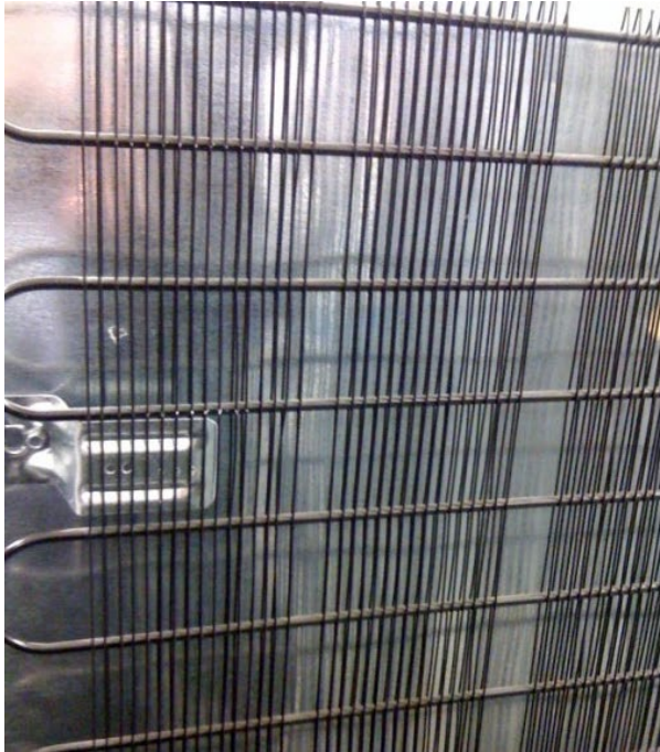
Standard back of the cabinet condenser Energy Star condenser packed under cabinet
