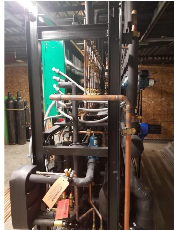
Sub-Cooling Only on Low Temperature System
