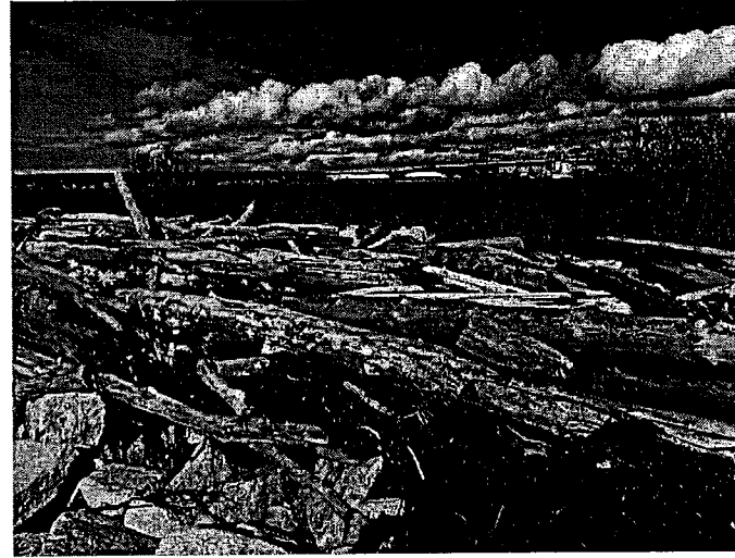
Wood on Top of Jetty
