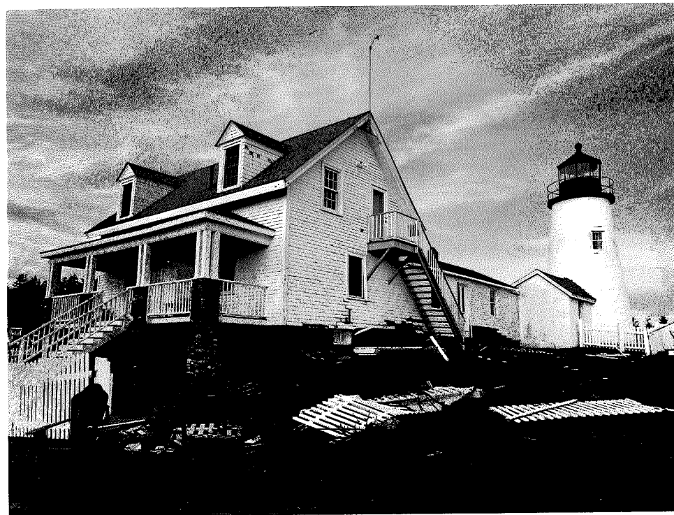
KEEPER'S HOUSE & FENCE
