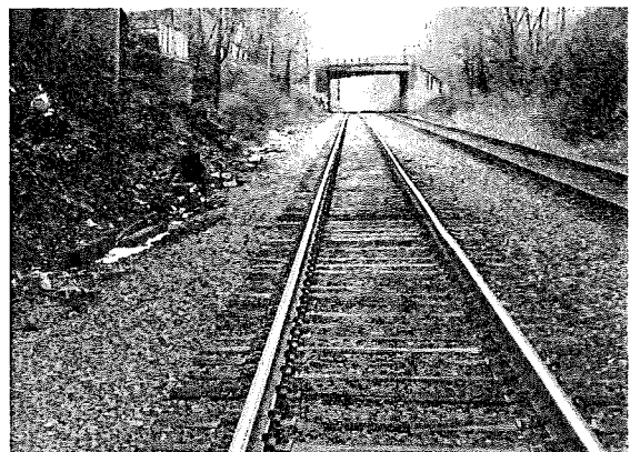
Figure 2-2: Class 5 Track (90 MPH Passenger)
