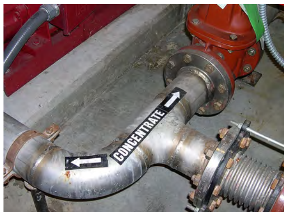
Fire suppression room, PFAS concentrate piping— a ticking time bomb Photo: Ed Friedman
