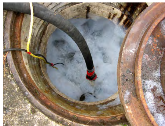
Sucking foam from sewer
