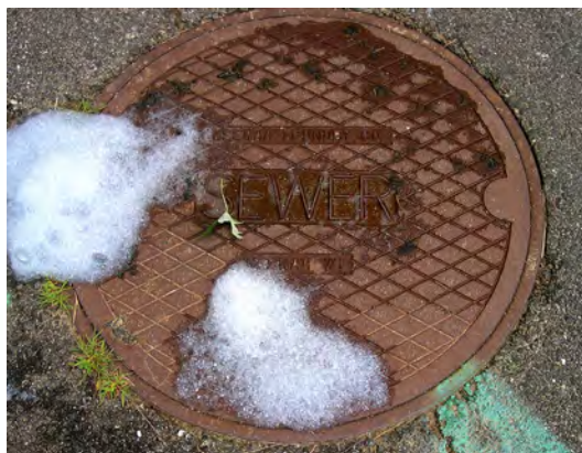
PFAS upwelling through the sewer manhole covers
