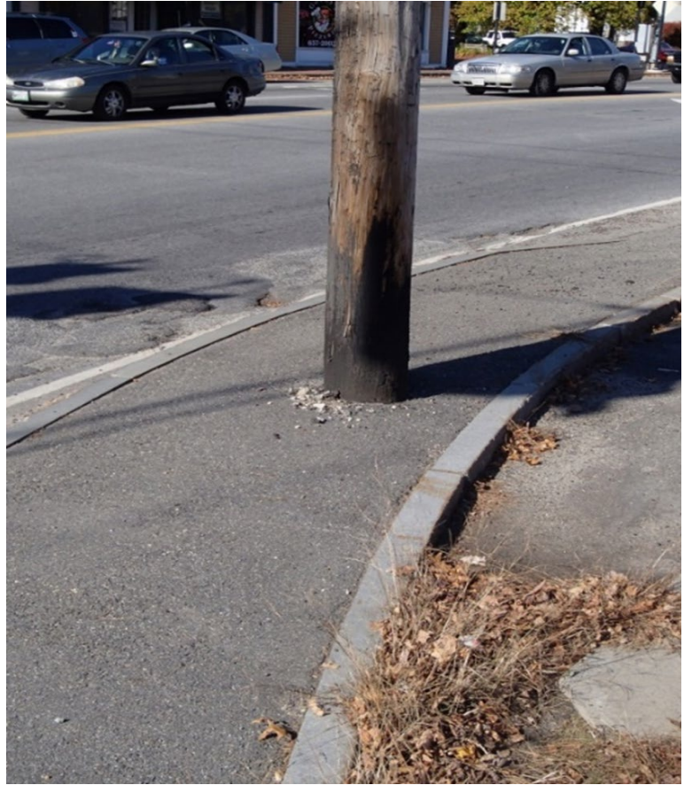
Figure 5: A wholly inadequate ramp and crosswalk on the corner of Main St. and Yarmouth Rd.
