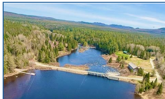
View of Churchill Dam, taken from a helicopter while inspecting harvest operations with the Maine Forest Service.
