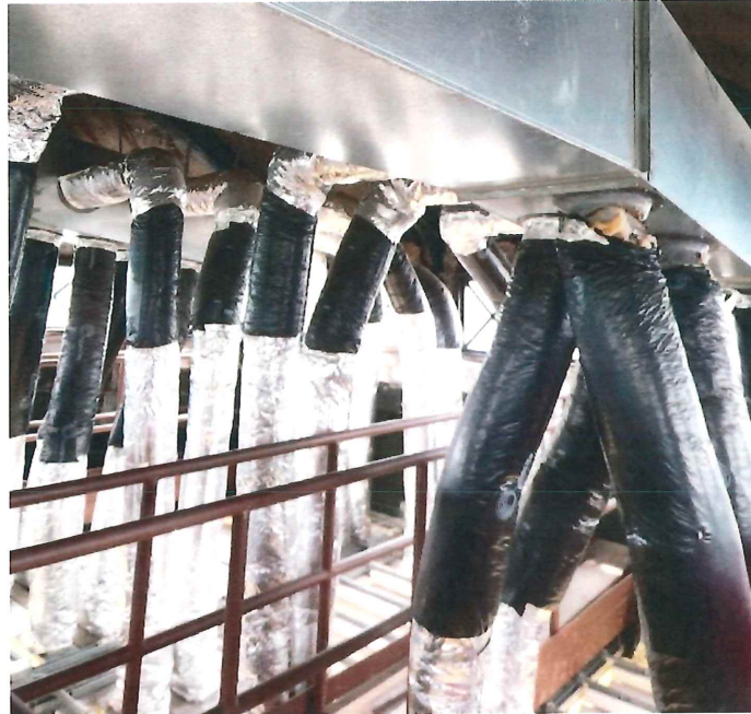
AHU-1 Supply Duct Distribution – North Shallow Dome
