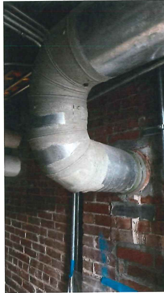
Typical Chimney Duct Connection.
