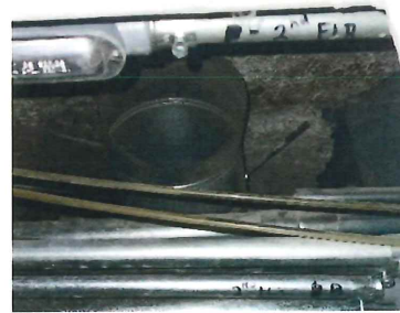
Open Duct in Attic
