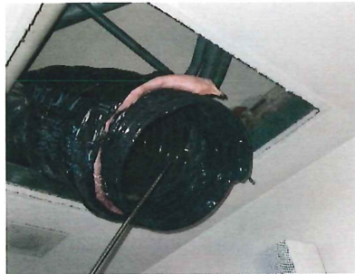
Open Duct Above Ceiling
