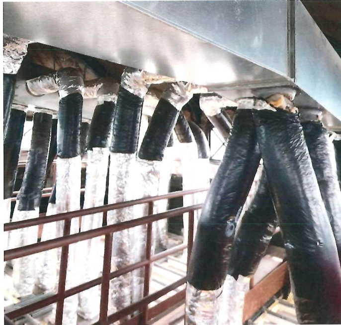
AHU-1 Supply Duct Distribution – North Shallow Dome
