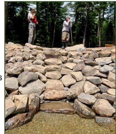
New stone steps at Scofield Point Campsite.
