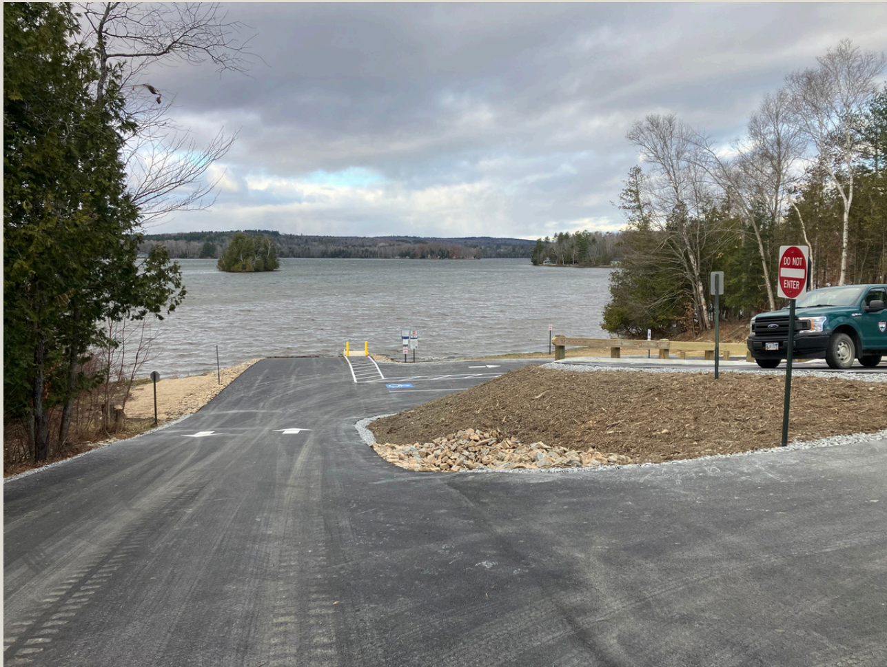
Big Indian Pond Water Access Site
